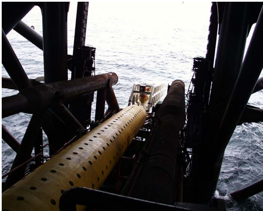
GRP Protection Tube during installation
